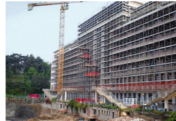
The restoration of the new SISSA Building.
