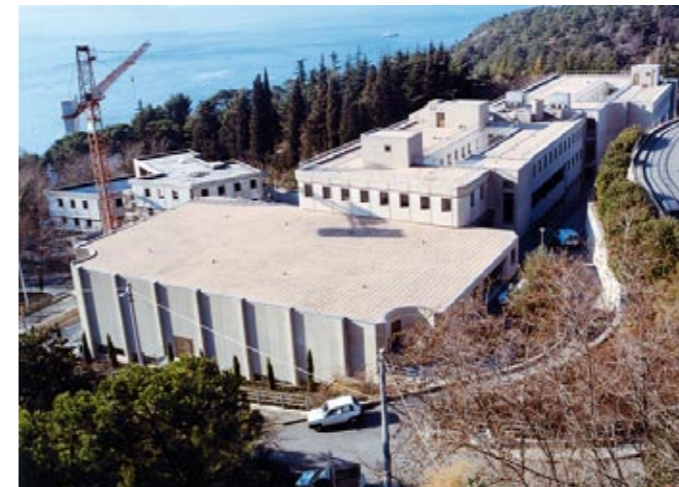
Construction of New Building.
